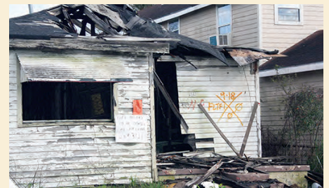
Markings in spray paint left by rescue workers are still visible on many structures in parts of New Orleans. They show the date the structure was searched, what organization performed the search, and how many people were found deceased in the home. Markings displaying "0" such as these meant all occupants made it out alive.
