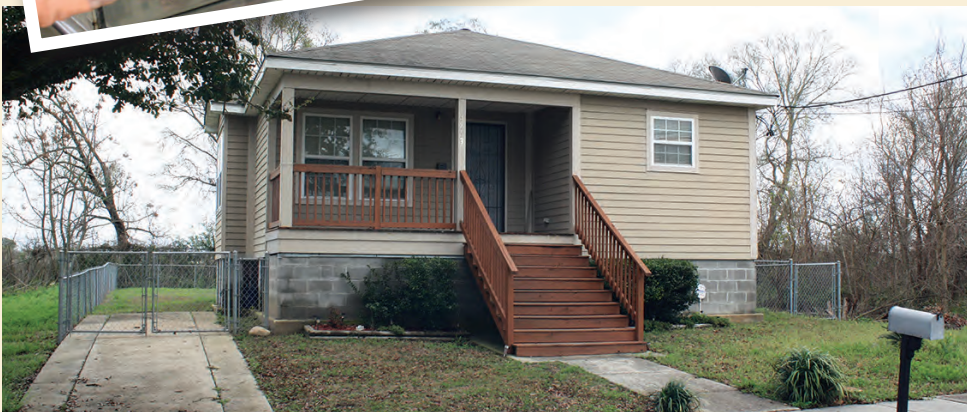
Once completed, the Habitat for Humanity Homes the students worked on will be very similar to this neighboring house.
