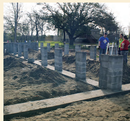
Throughout much of New Orleans, the water table sits just a foot below the ground's surface. For this reason, homes here have no basements, and foundations are made out of columns of cement blocks, and filled with mixed cement for reinforcement.
